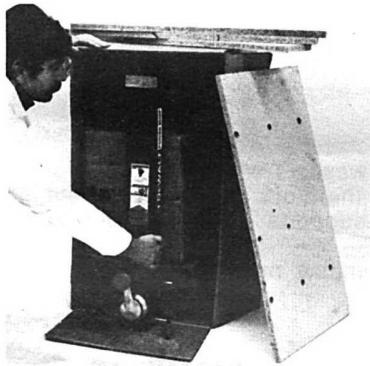
1. Remove guard box and all loose packing, tip carton on end and remove machine.
